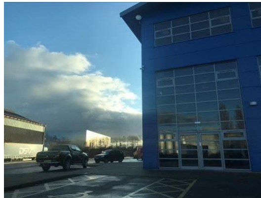
Tinsley Park occupied by Tinsley Bridge Group Engineering Solutions
