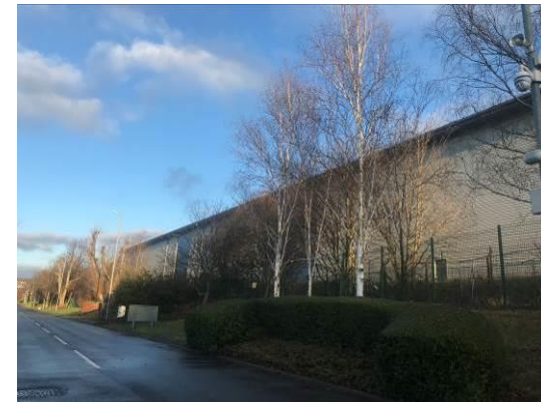
Tinsley Park occupied by Tinsley Bridge Group Engineering Solutions
