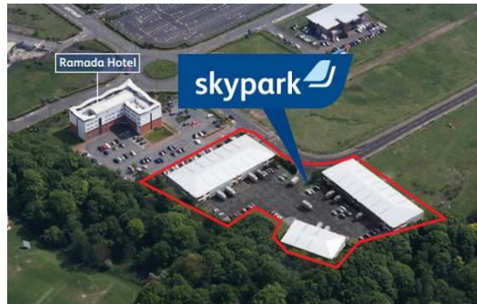
RHAD - Aerial of Skypark
